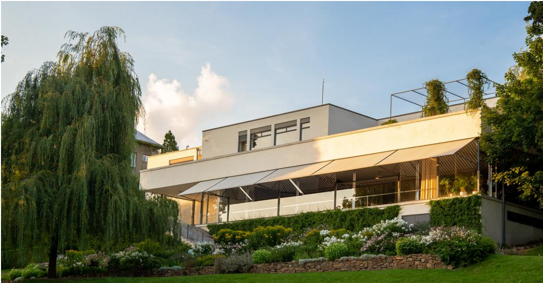
Villa Tugendhat: the white horizontal element, above a wall of glass, floats above a flower bed
