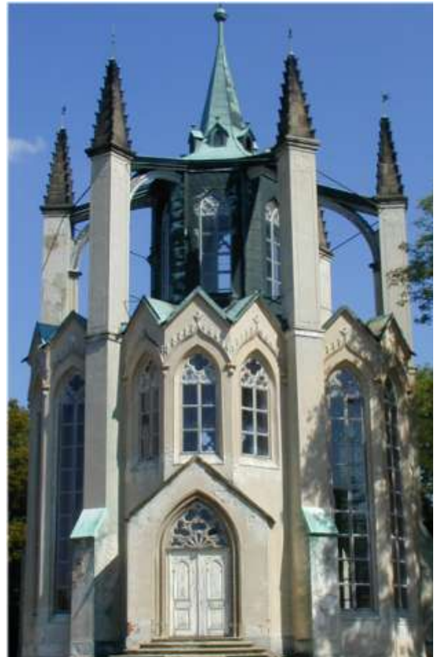
Krásný Dvůr, The Park The Gothic Temple Left, a section showing the staircase arrangement, taken from the original plan of 1792. Below, an exterior view today
