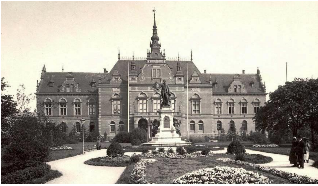
Left, the German House in Brno in 1900, demolished in 1945.
